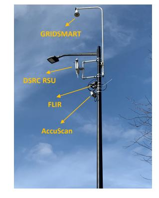
Long range sensors: AccuScan radar sensors and FLIR thermal image sensors
